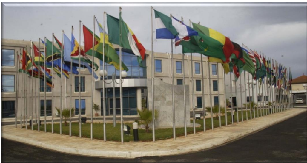
ACSRT OFFICES - ALGIERS
